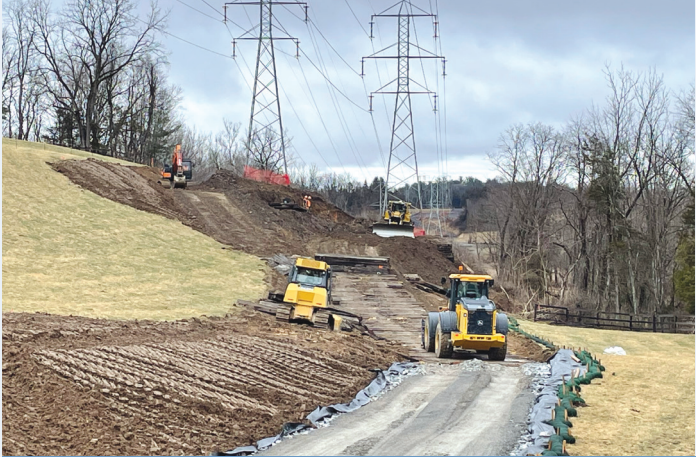
The photo at left shows a portion of the NYES corridor as our crews prepared to remove the existing lattice structures. At right is the same location today with the new monopoles in place and site restoration underway.
